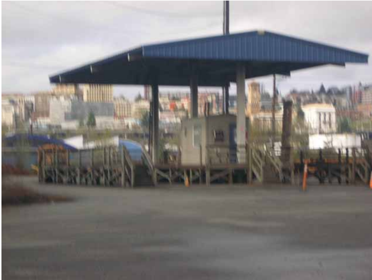
Some racks are covered.
