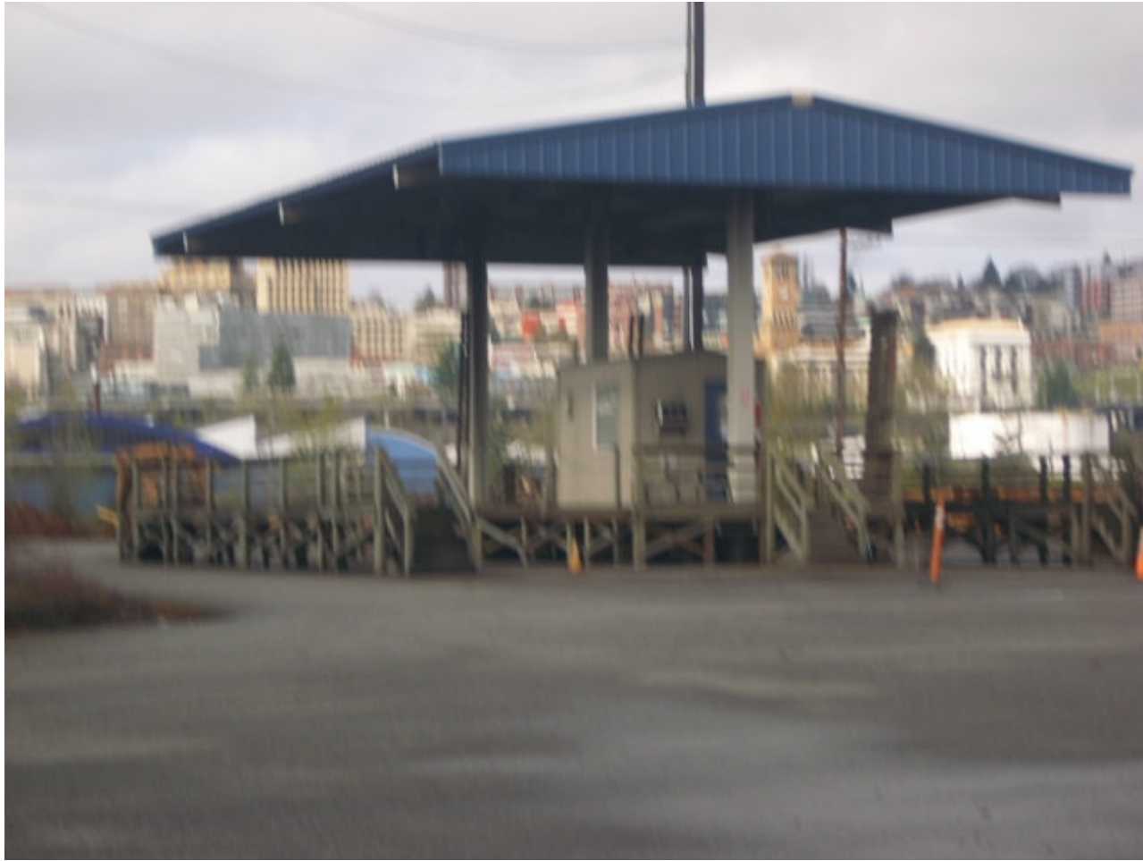
Some racks are covered.
