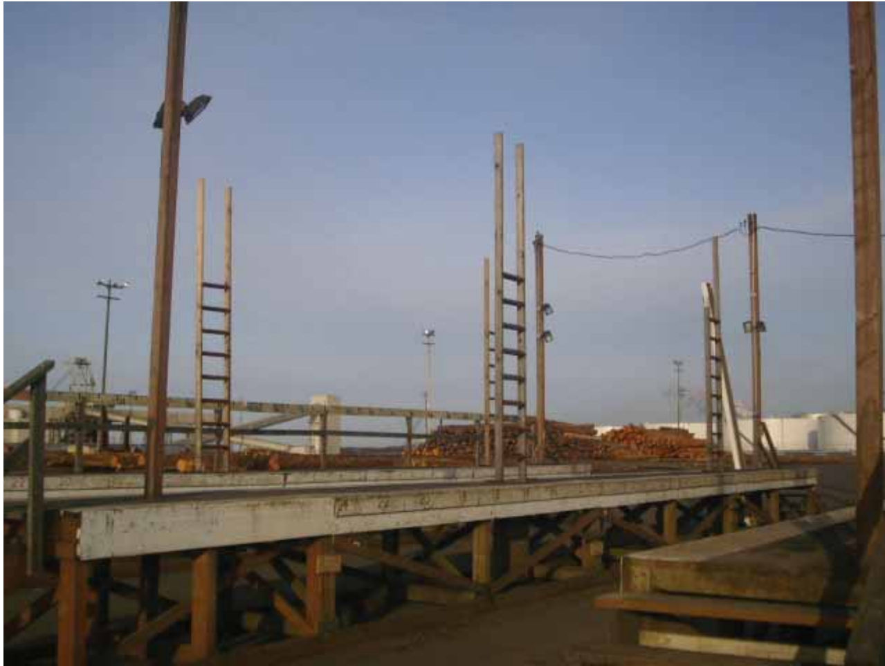
Each scale bay has 4 ladders, 2 on each side of the load.
