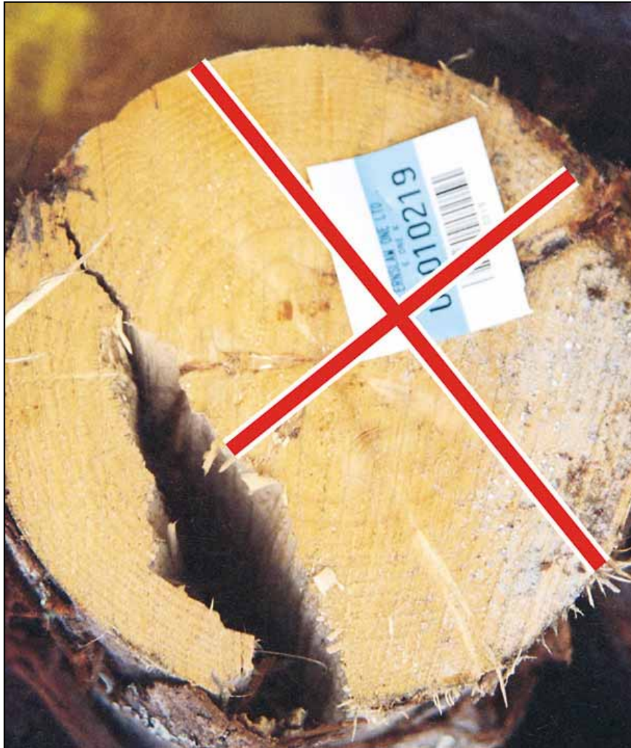
Fig. 27: Broken end. Exclude broken piece because it extends more than 10 cm into the log.
